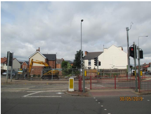
The application site. 4 Waverley Avenue to the left, and 198 Station Road to the right
