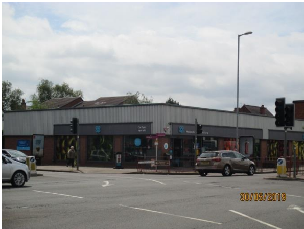
The Co-op supermarket opposite the site
